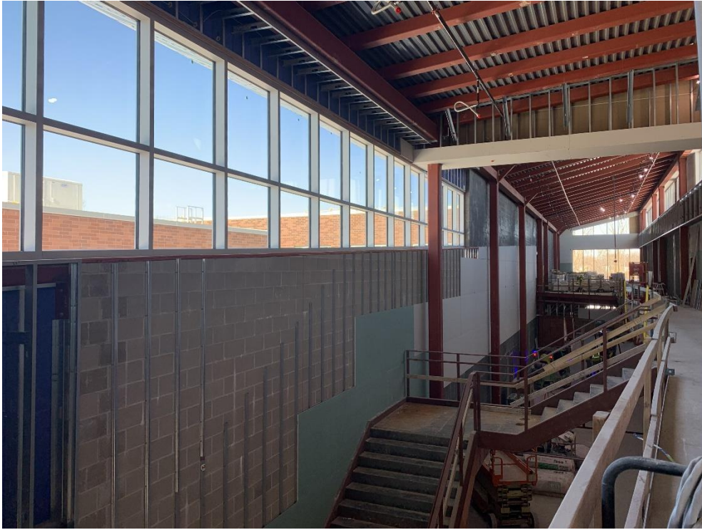
36. Area 1A – Above ceiling MEP and gyp board install in progress at LMC.
