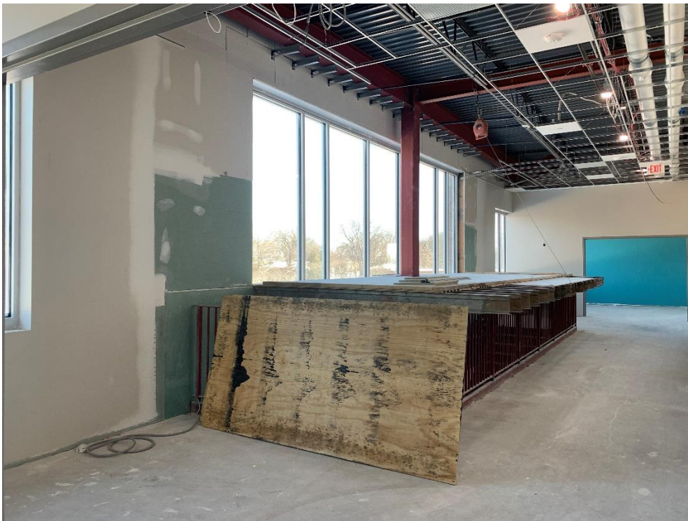
18. Area 5 – Gyp board install, taping, and mudding at north stair in progress. Ceiling grid install continues.
