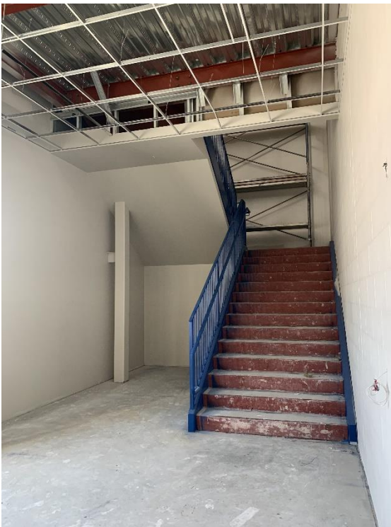
8. Area 5&6 – Gyp board finishing, painting, and ceiling grid install at stairs in progress.
