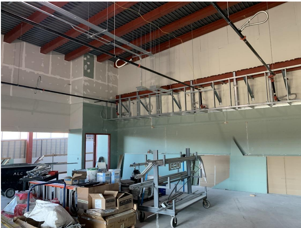
38. Area 1A – Gyp board install, taping, and mudding at second floor community room in progress.
