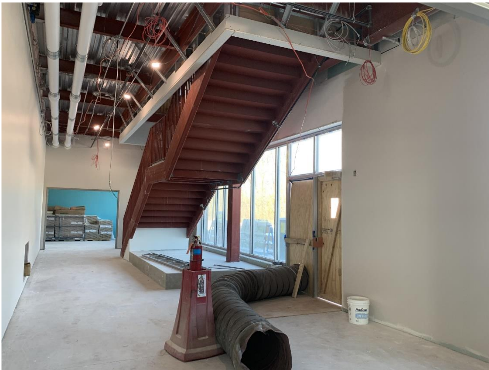
22. Area 5 – First floor gyp board soffit install and painting at north stair in progress.
