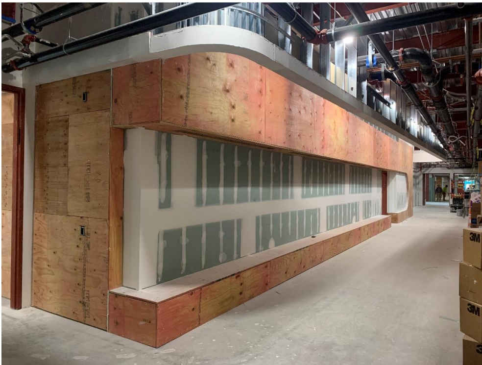
26. Area 4 – Plywood backing install, gyp board taping and mudding of first floor gradewalling entry feature in progress.
