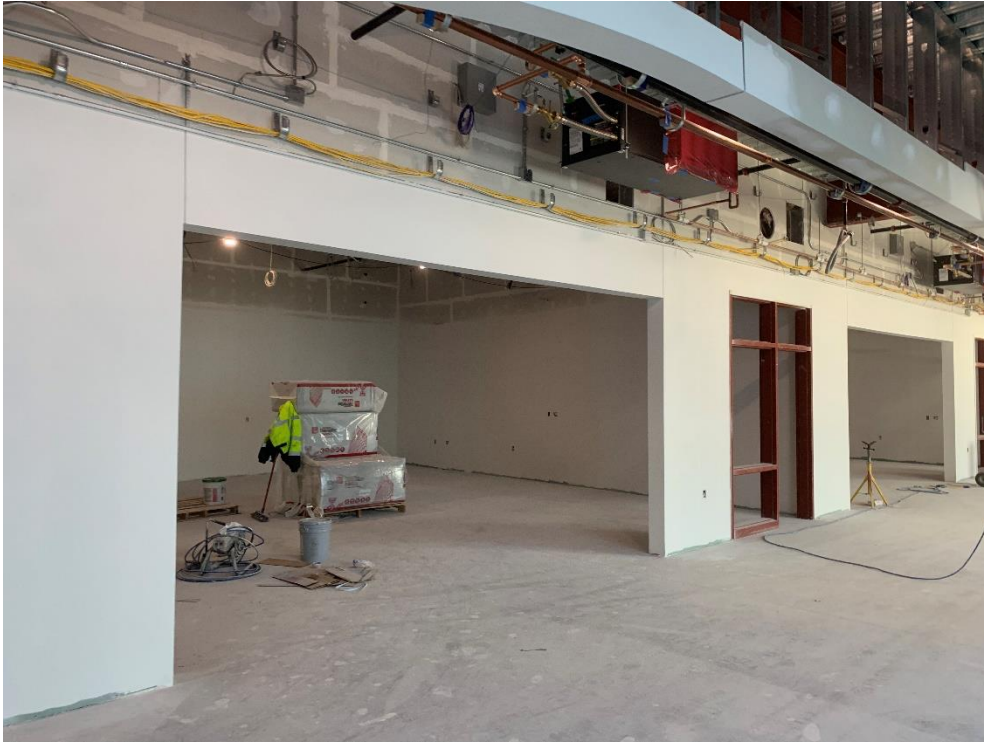
26. Area 4 – Plywood backing install, gyp board taping and mudding of first floor gradewalling entry feature in progress.
