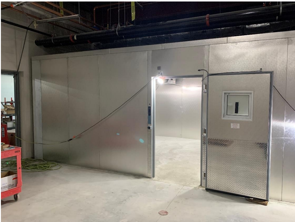
40. Area 3 – Cooler and freezer install at production kitchen in progress.
