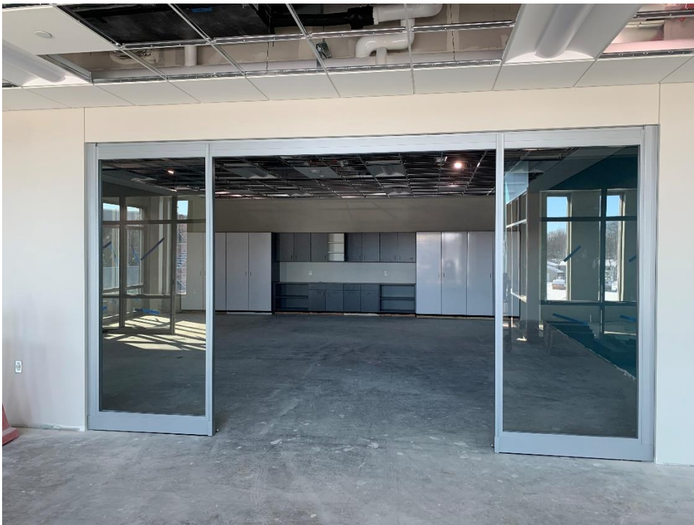
16. Area 5 – Casework and glass sliding door system install in second floor classrooms in progress.
