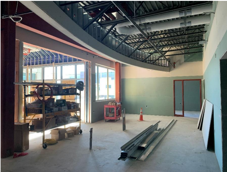
48. Area 1A – Gyp board install, taping, mudding, and above ceiling MEP work in progress at 5/6 front office.
