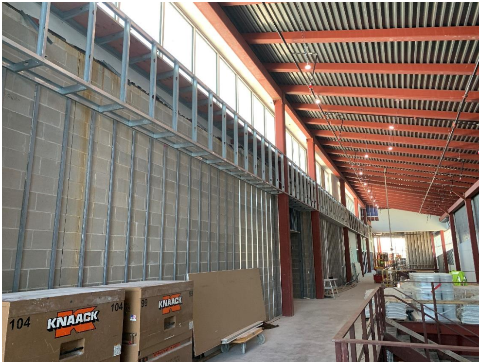
34. Area 1A&B – Center spine guard rail metal frame install in progress.
