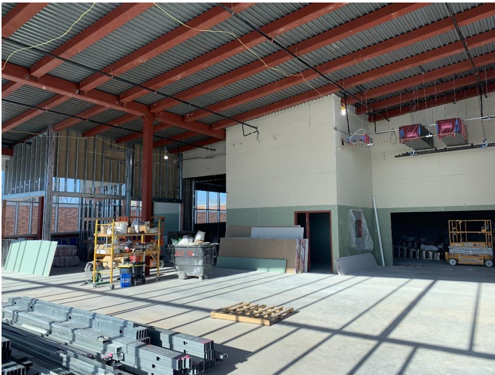
36. Area 1A – Above ceiling MEP and gyp board install in progress at LMC.
