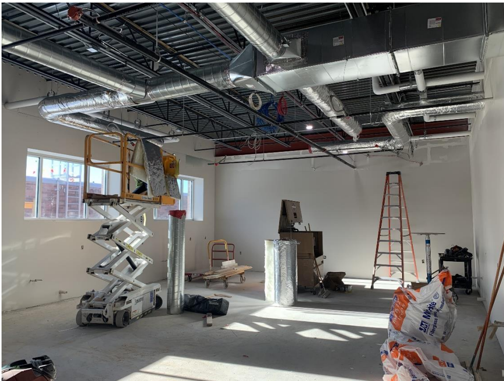
32. Area 3 – Above ceiling MEP work and duct insulation install in progress at second floor art rooms.
