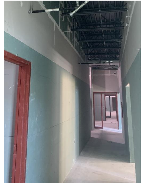
48. Area 1A – Gyp board install, taping, mudding, and above ceiling MEP work in progress at 5/6 front office.
