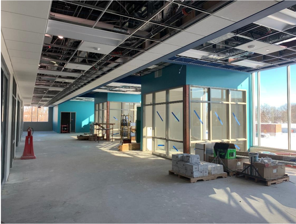
18. Area 5 – Gyp board install, taping, and mudding at north stair in progress. Ceiling grid install continues.
