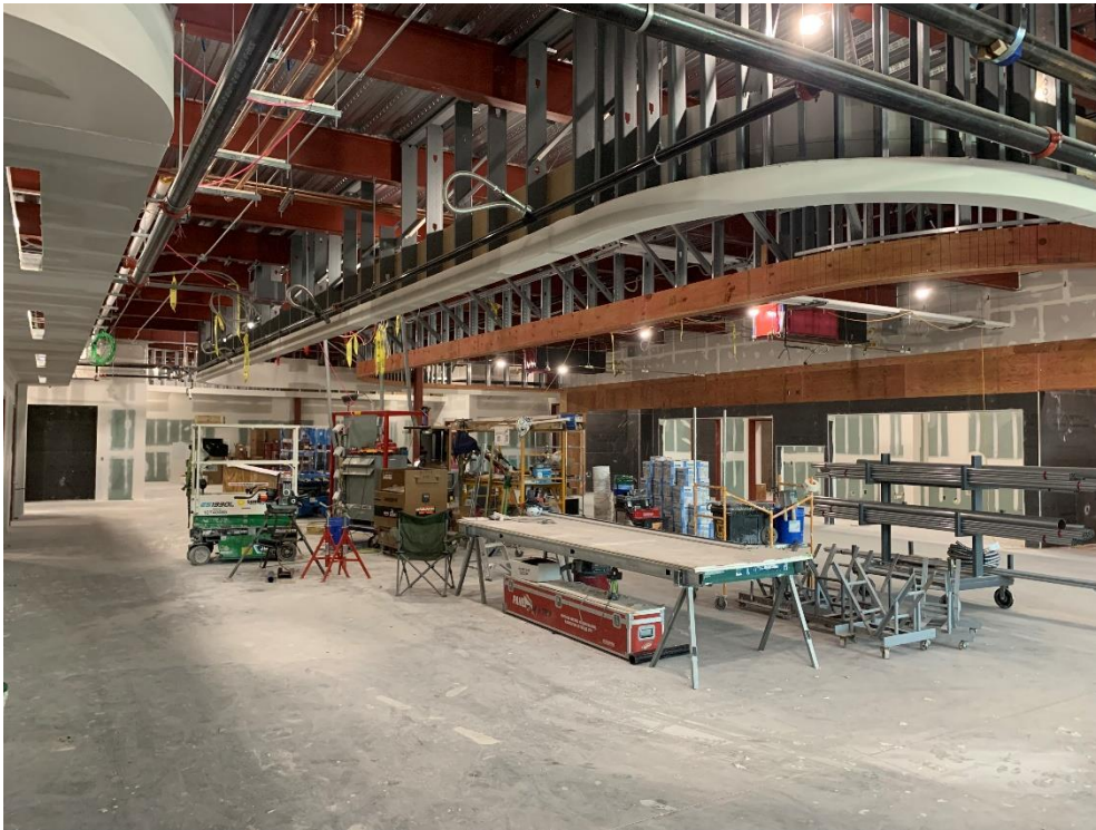
24. Area 4 – Gyp board taping, mudding, and painting at first floor collab areas and classrooms in progress.
